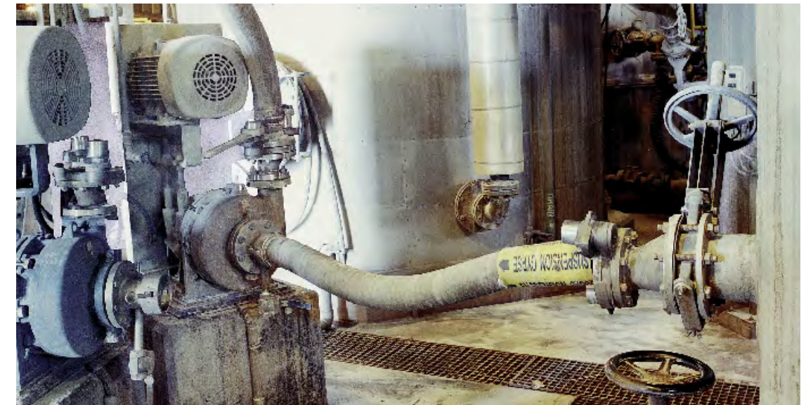
An industrial installation is shown above. RITE CAMLOCK COUPLINGS allow the user to rapidly disconnect the hose from the storage tank and connect it to another. Also the hose can be connected with a RITE CAMLOCK COUPLING to the pump as shown below.
