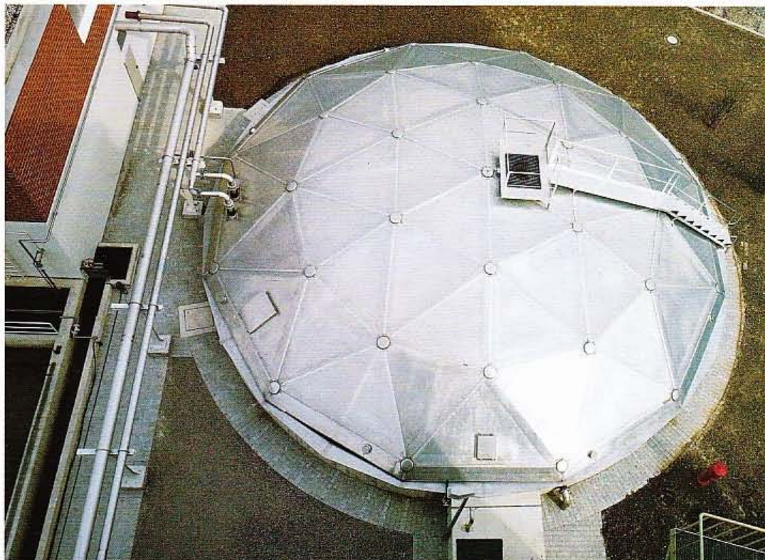
VACONODOME® 16,8 m diameter covering an aeration tank
