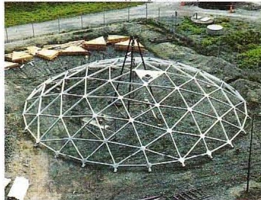
VACONODOME® 19,5 m diameter covered with prefabricated sheets
